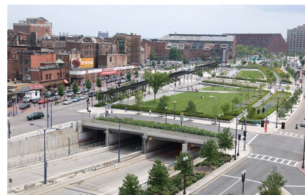
SOME ROADS GO THROUGH TUNNELS
