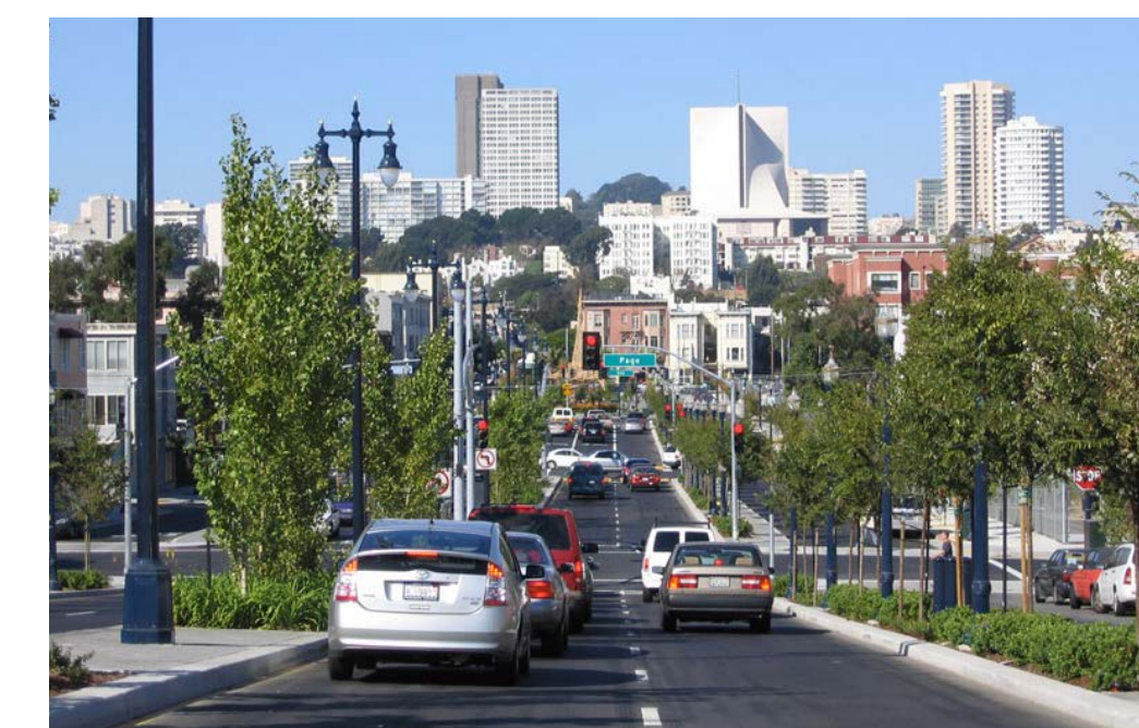
SOME ROADS ARE 'AT GRADE'
